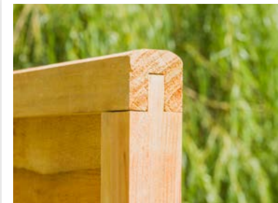
Superior Lap, mortice and tenon joint
